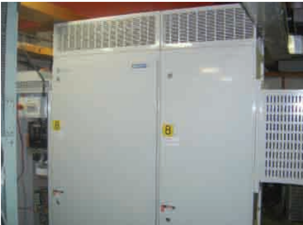
Top: A Quattro controller in the Northbank Plaza's high-rise machine room, along with an Otis E413M machine. An old Schindler Miconic V12 Pulse DC controller is in the background.
