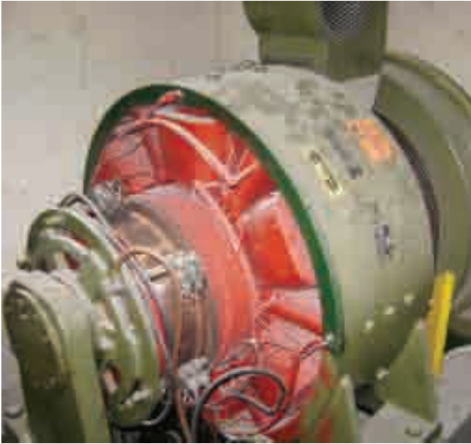
A close-up view of an Otis 155HT hoist motor in the Northbank Plaza's low-rise machine room
