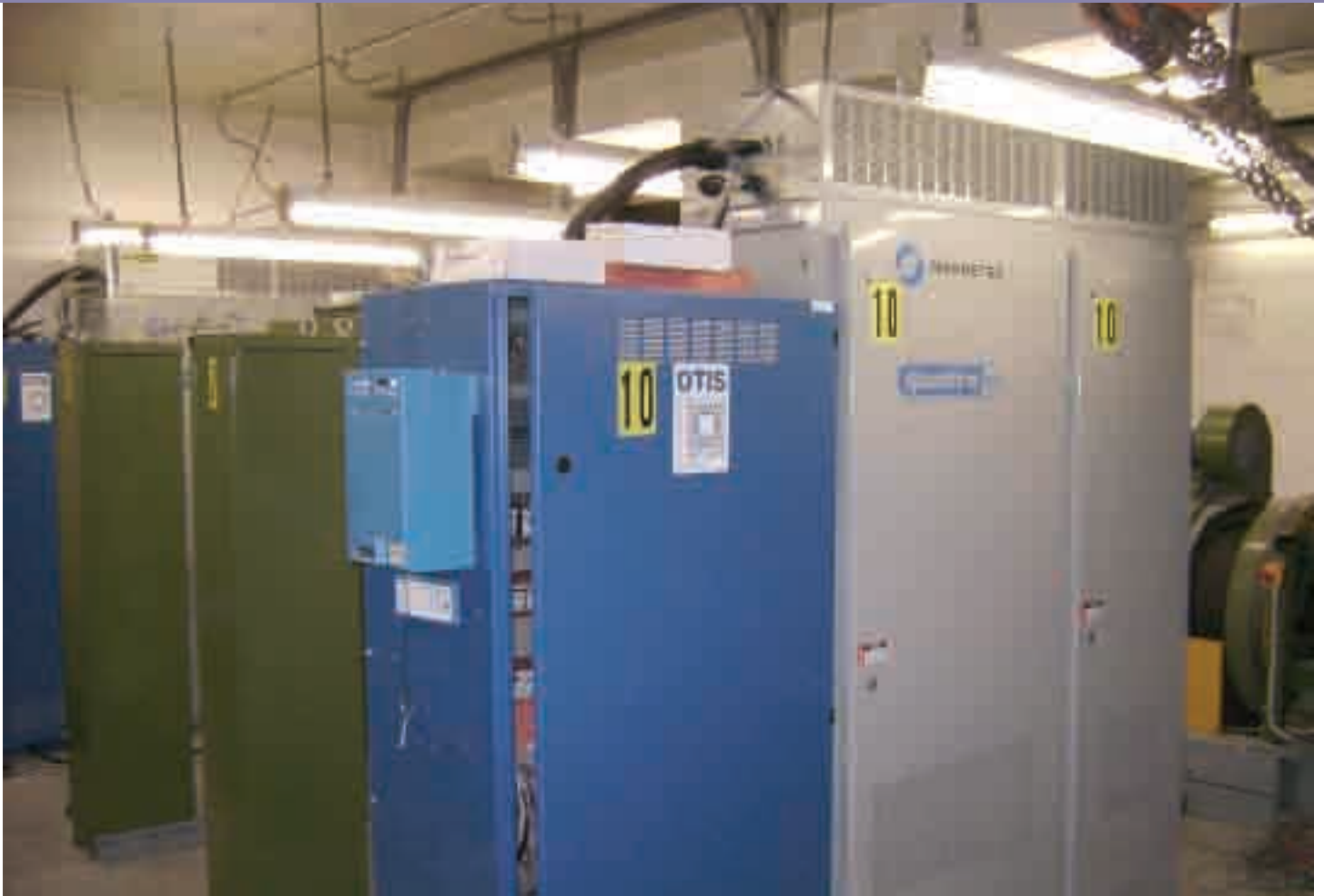
Top: A Quattro controller in the Northbank Plaza's high-rise machine room, along with an Otis E413M machine. An old Schindler Miconic V12 Pulse DC controller is in the background.
