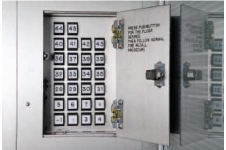
*Floor buttons are located behind a locked cabinet in the car-operating panel. This opens automatically during an emergency for access by firefighters.*
