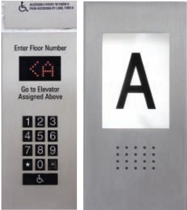
Top left: The destination-dispatch elevator-system keypad that directs passengers to the correct elevator
