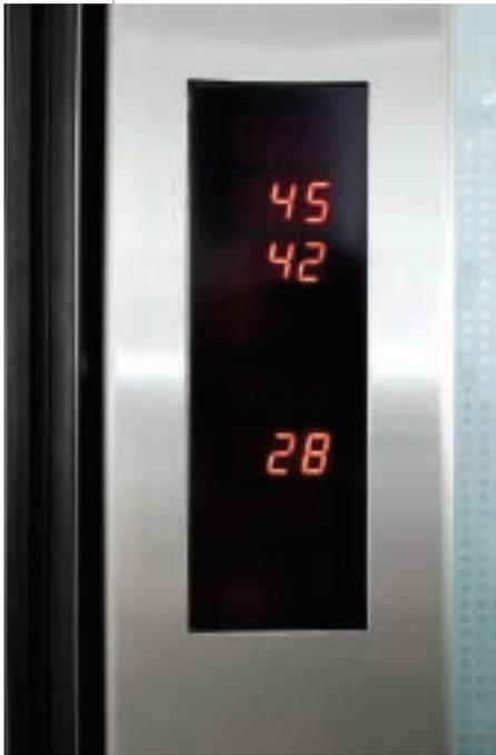
The in-car destination indicator, next to the elevator doors, indicates the floors at which the car will make stops.
